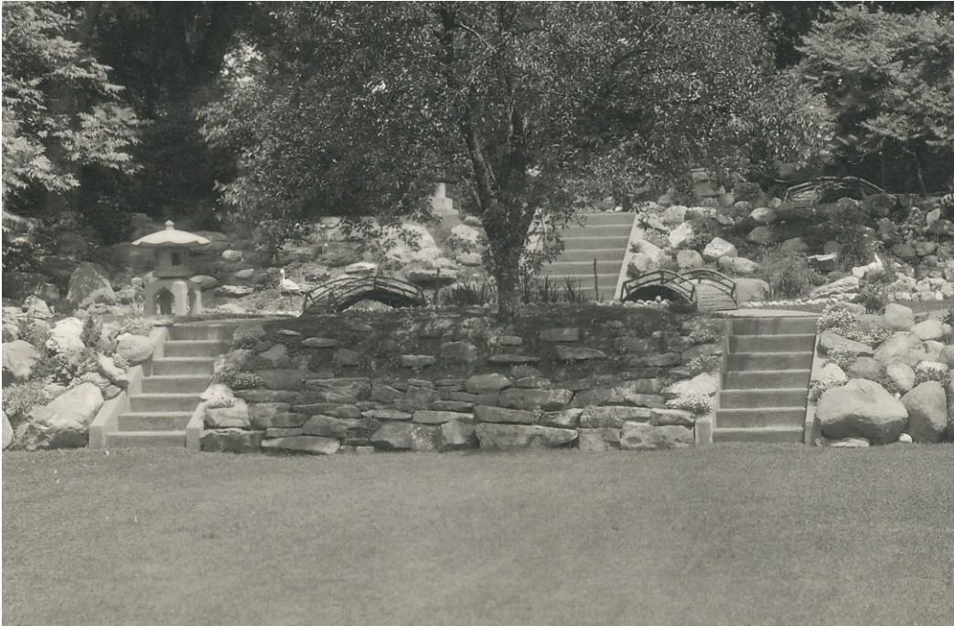
Figure 77: The center section of the bottom slope of Mrs. McColm's garden was constructed with a stacked horizontal pattern (unlike the other sloping sections of rounded rocks and boulders – maybe Mrs. McColm liked the look of both the stacked pattern and the more natural boulders and wanted both). The center rocks were not as uniformly flat as those used for the shrine steps, perhaps because thicker stones were deliberately used at the bottom for visual weight. (MAC)
