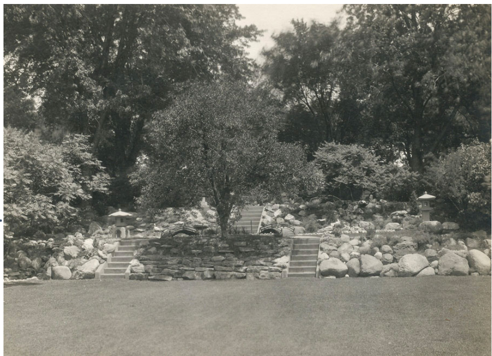
Figure 36: This photo shows the three levels of the Japanese garden. Boulders are arranged to anchor the changes in grade between the levels, with a different stacked limestone arrangement in the lower center section. (MAC)
